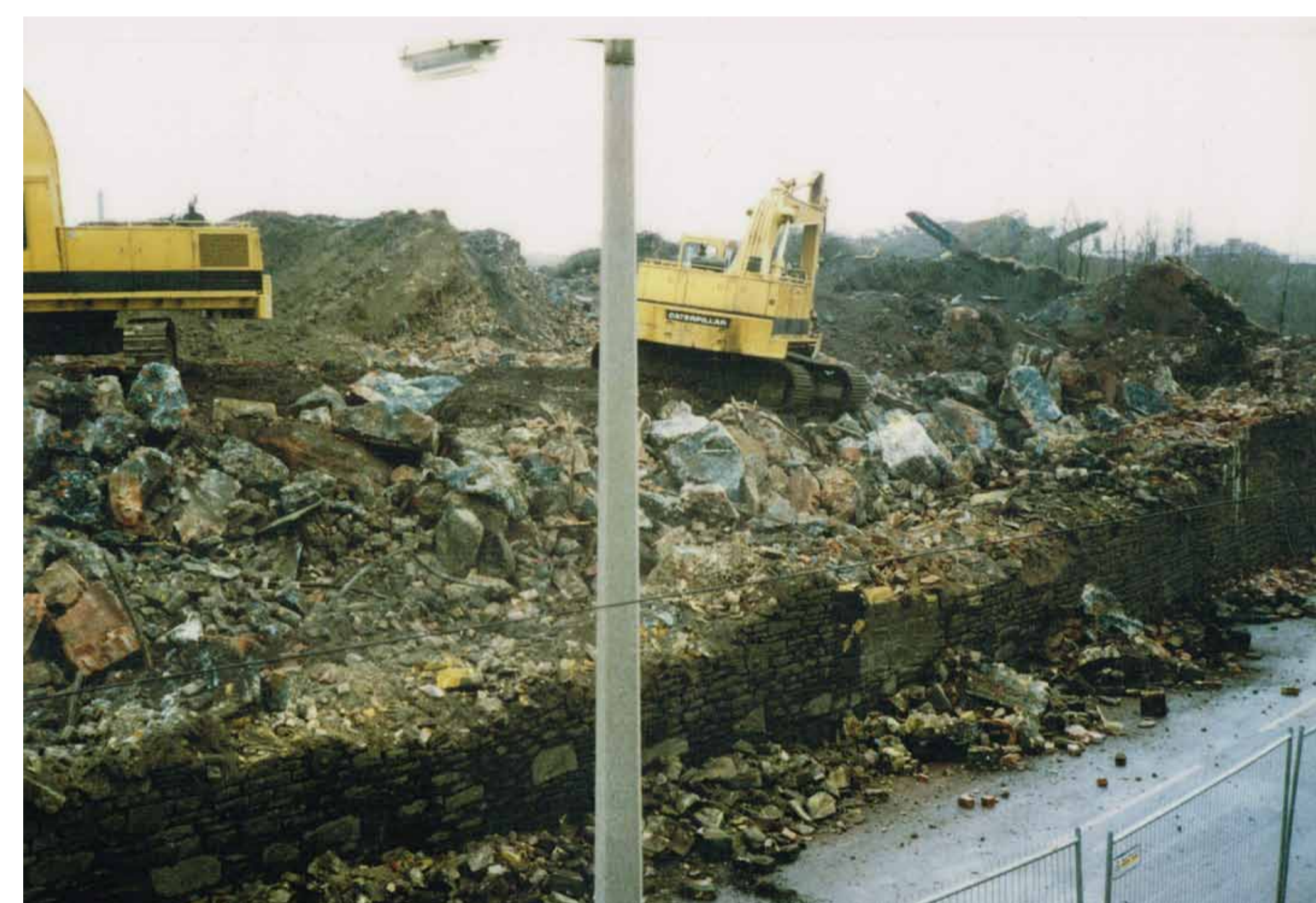
View from site side of wall Showing height of wall after work had started on lowering wall to daylight to blomas
