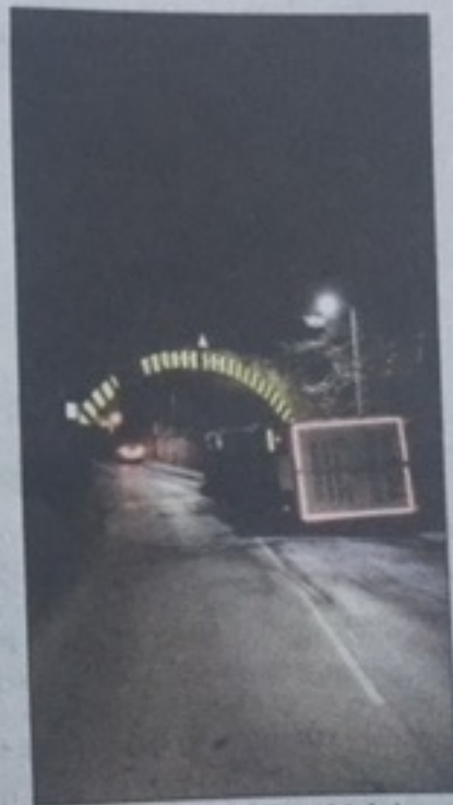
bridge at Springvale, which is one of several in the area with a history of collisions involving lorries.
